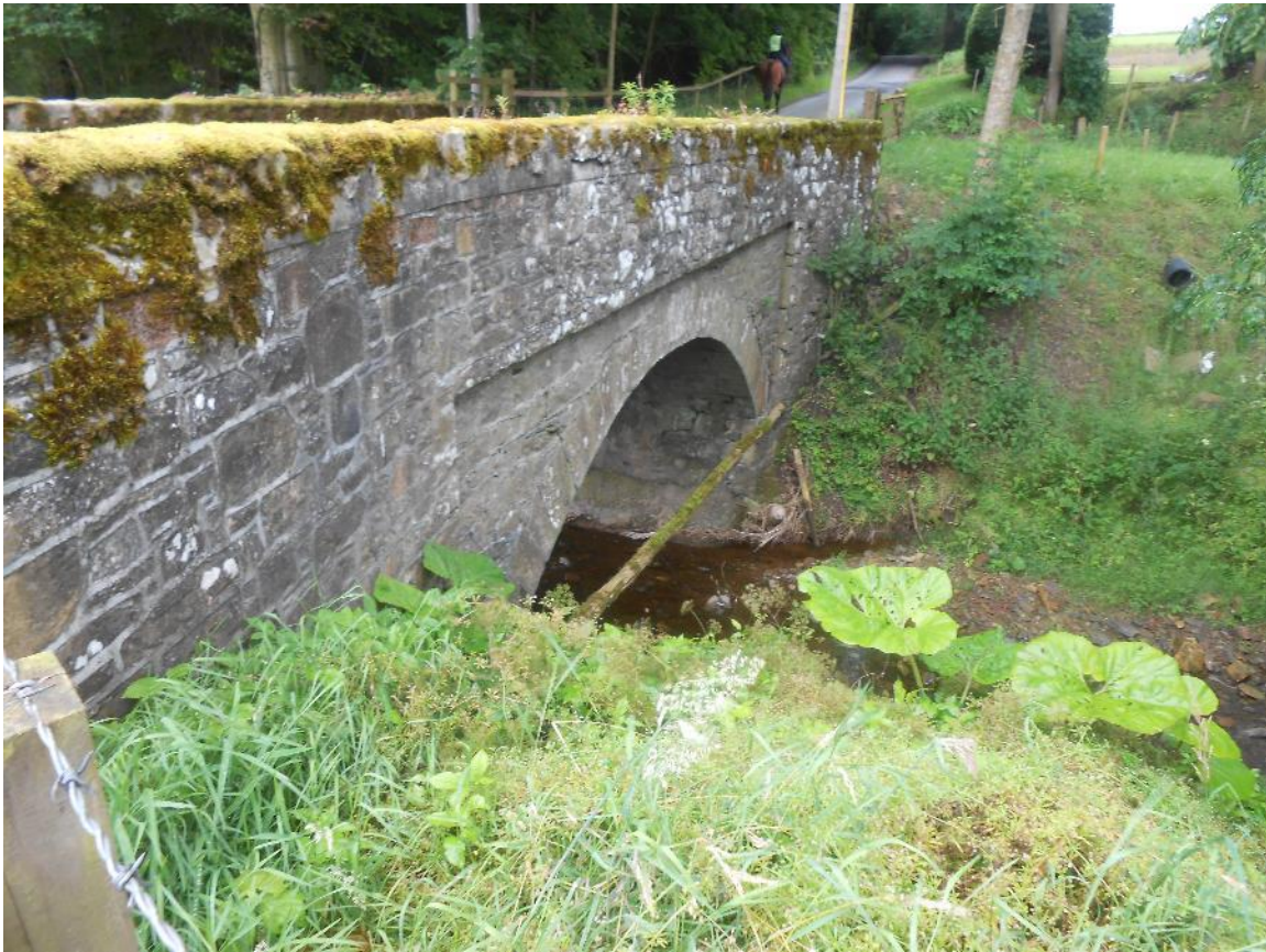
Photo 5: B6357 road bridge (view from upstream side)
